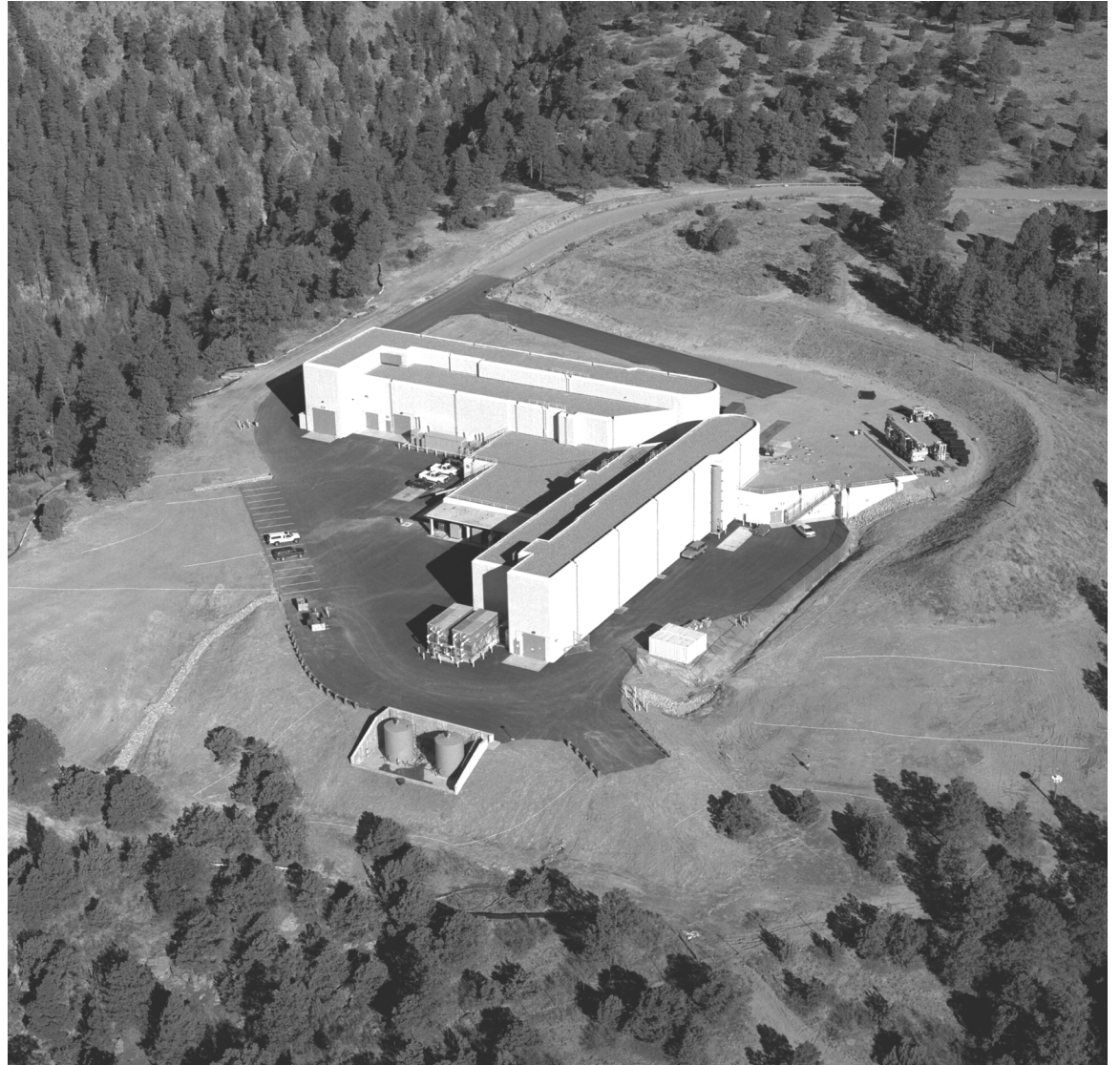
Figure IV-3: Alternate view of DARHT facility
